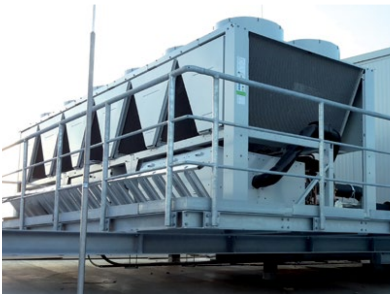
750 kW cold brine unit with screw-type compressor and heat recuperation
